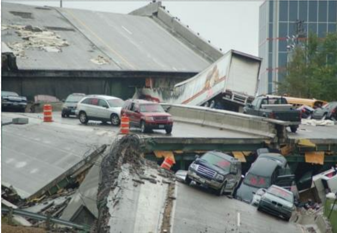
I-35W Bridge in Minneapolis, Minnesota suddenly collapsed during the evening rush hour, in 2007.
