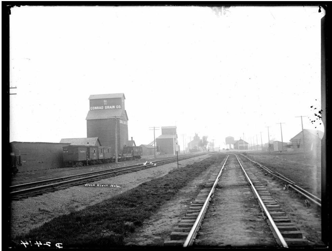
Figure 3 - Elevators at Wood River, Nebraska, circa 1910, Nebraska State Historical Society
