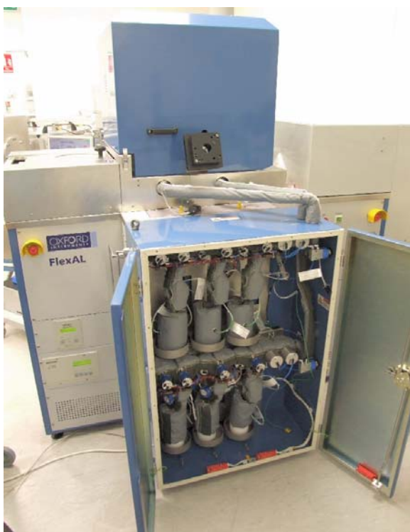
Figure 2-21 General view of the six-way precursor cabinet
