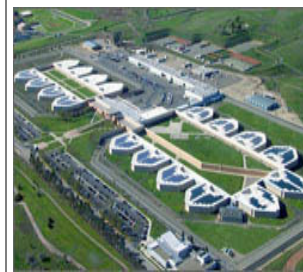
In Spring 2002, largest solar electric system in the US began operating atop the Santa Rita Jail in Dublin, California. This solar installation, helps Alameda County reduce and stabilize energy costs.
