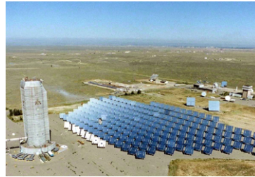
At the National Solar Thermal Test Facility (NSTTF) , built at Sandia National Laboratories in Albuquerque in 1976, the 63-meter tall tower has 222 computer-controlled heliostats that can direct the sun into any of four test bays to produce a total thermal capacity of 5 megawatts.
