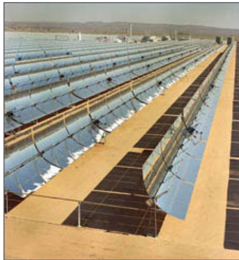
Solar thermal power plant. (Mojave Desert in Kramer Junction, California) This is one of nine such plants built in the 1980s. During operation, oil in the receiver tubes collects the concentrated solar energy as heat and is pumped to a power block (in background) for generating electricity.
