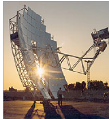
Solar dish-engine system. The dish, a concentrator, collects the energy coming directly from the sun and concentrates it on a small area. A thermal receiver absorbs the concentrated beam of solar energy, converts it to heat, and transfers the heat to the engine/generator. (Credit: Sandia National Laboratories)
