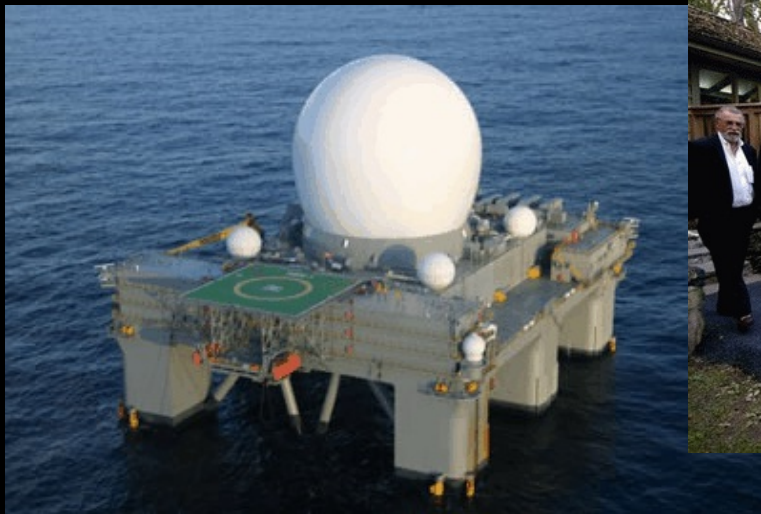
X-Band Radar Installation in the Pacific
