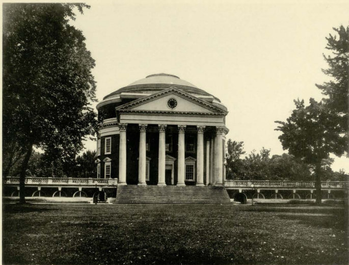
RESTORATION OF ROTUNDA & TERRACES ACCORDING TO THE ORIGINAL SCHEME OF THOMAS JEFFERSON, ARCHITECT.
