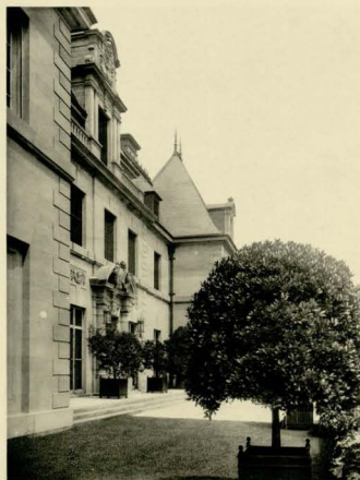
TERRACE AT ENTRANCE
