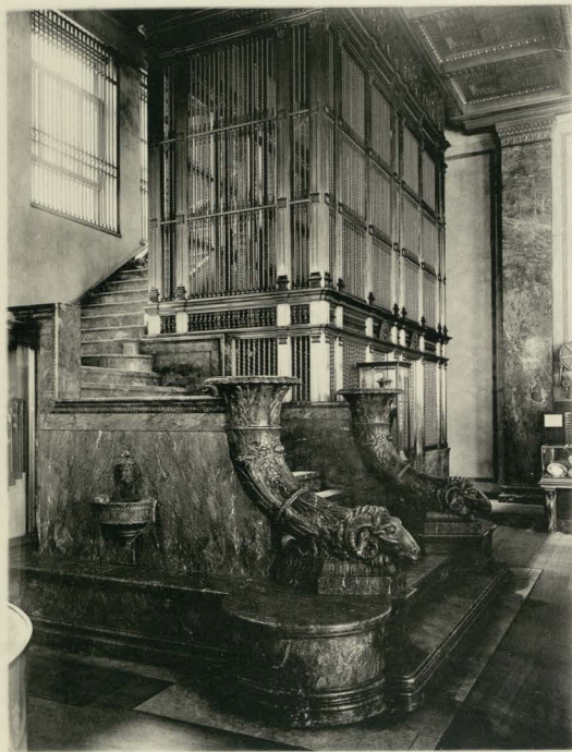
STAIR AND ELEVATOR ENCLOSURE
