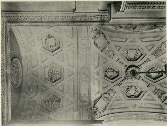
CEILING OF LOGGIA
