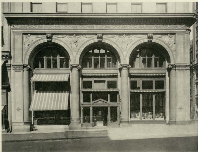
EXTERIOR DETAILS BUILDING FOR THE GORHAM COMPANY, NEW YORK CITY. 1906
