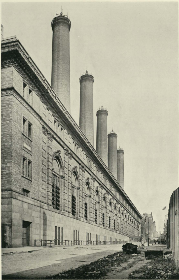
INTERBOROUGH RAPID TRANSIT COMPANY, NEW YORK CITY POWER HOUSE 1903
