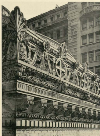
DETAIL OF UPPER CORNICE
