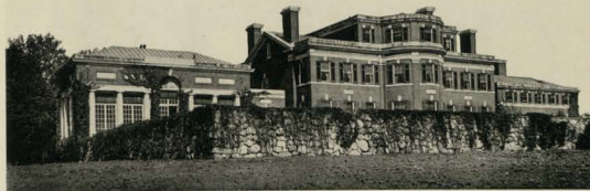
FACADE FACING SEA
