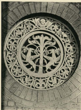
DETAIL OF ROUND WINDOW UNDER PORTICO
