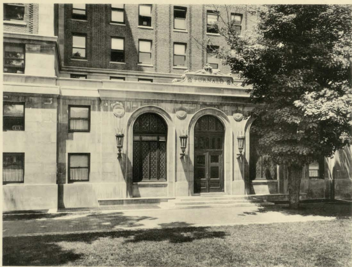
FURNALD HALL, DORMITORY, 1912
