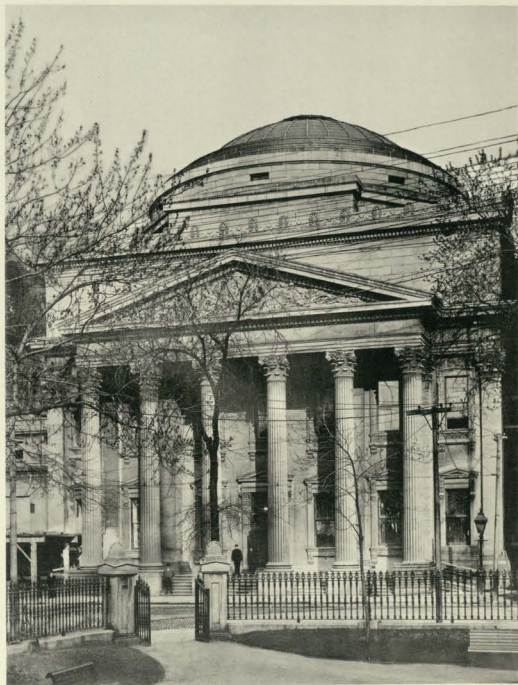
ST. JAMES STREET FACADE
