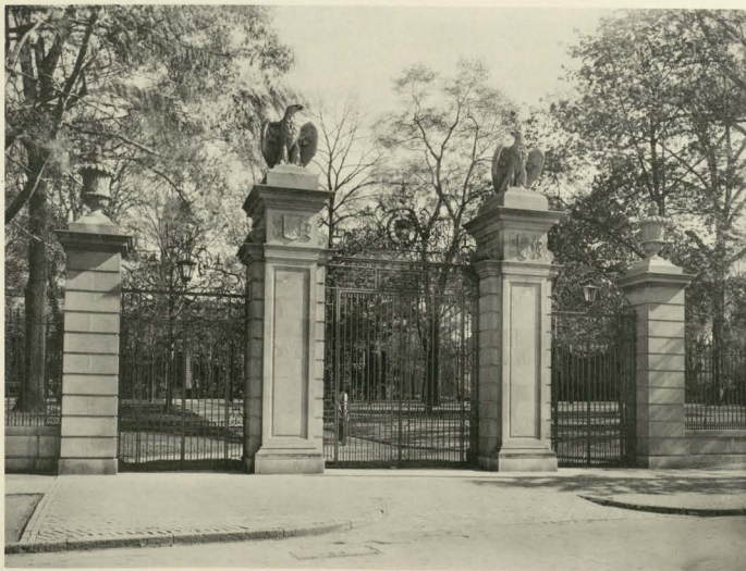
MAIN ENTRANCE GATES, NASSAU STREET - 1905
