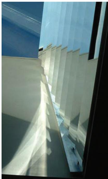
Detail of a skylight designed to redirect and optimize daylight in Marilyne Andersen’s MIT office. The assembly includes aluminum slats of varying inclination angles that maximize daylight penetration into the office space while avoiding reflections on the computer screen—and creating interesting visual effects.
