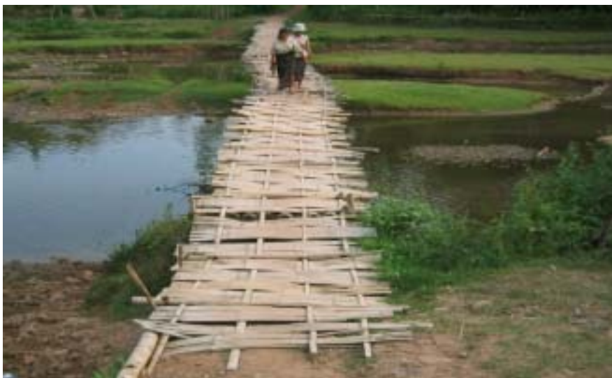
Figure 3.2: Bamboo Footbridge with Pier Support
