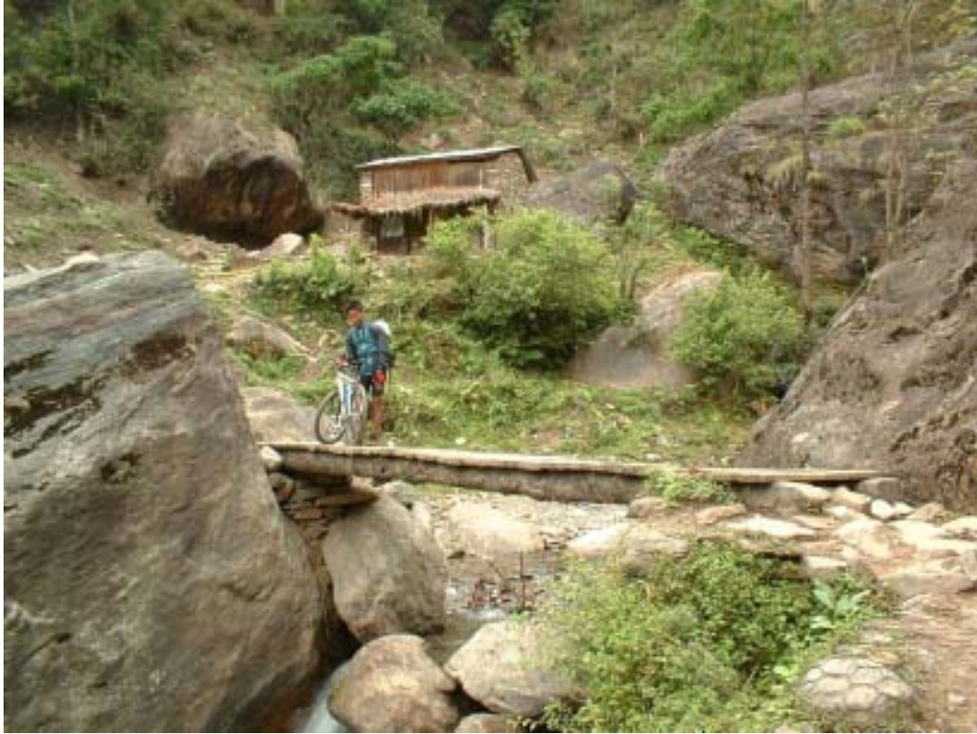
Figure 4.9: Basic Timber Log Footbridge in Nepal
