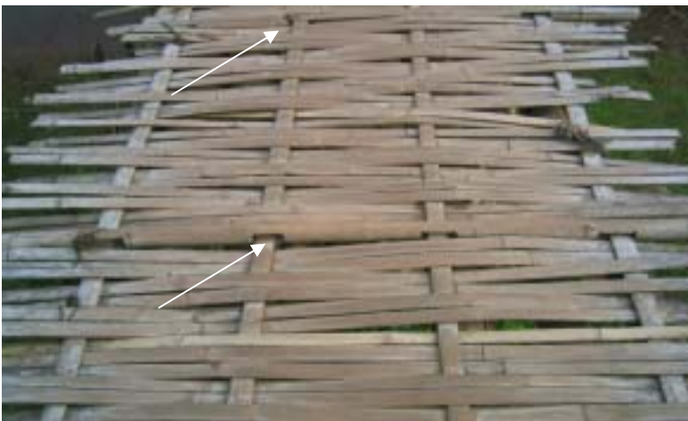
Figure 4.2: Details of a Simple Bamboo Footbridge from Laos
