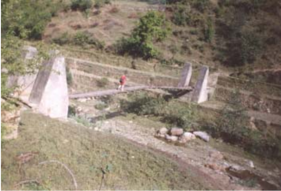
Figure 3.15: 30m Span Suspension Footbridge in Nepal
