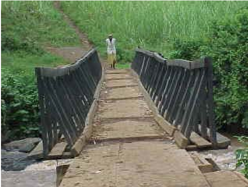
Figure C1: Footbridge Using a Scrap Truck Chassis for the Beams Supporting the Deck
