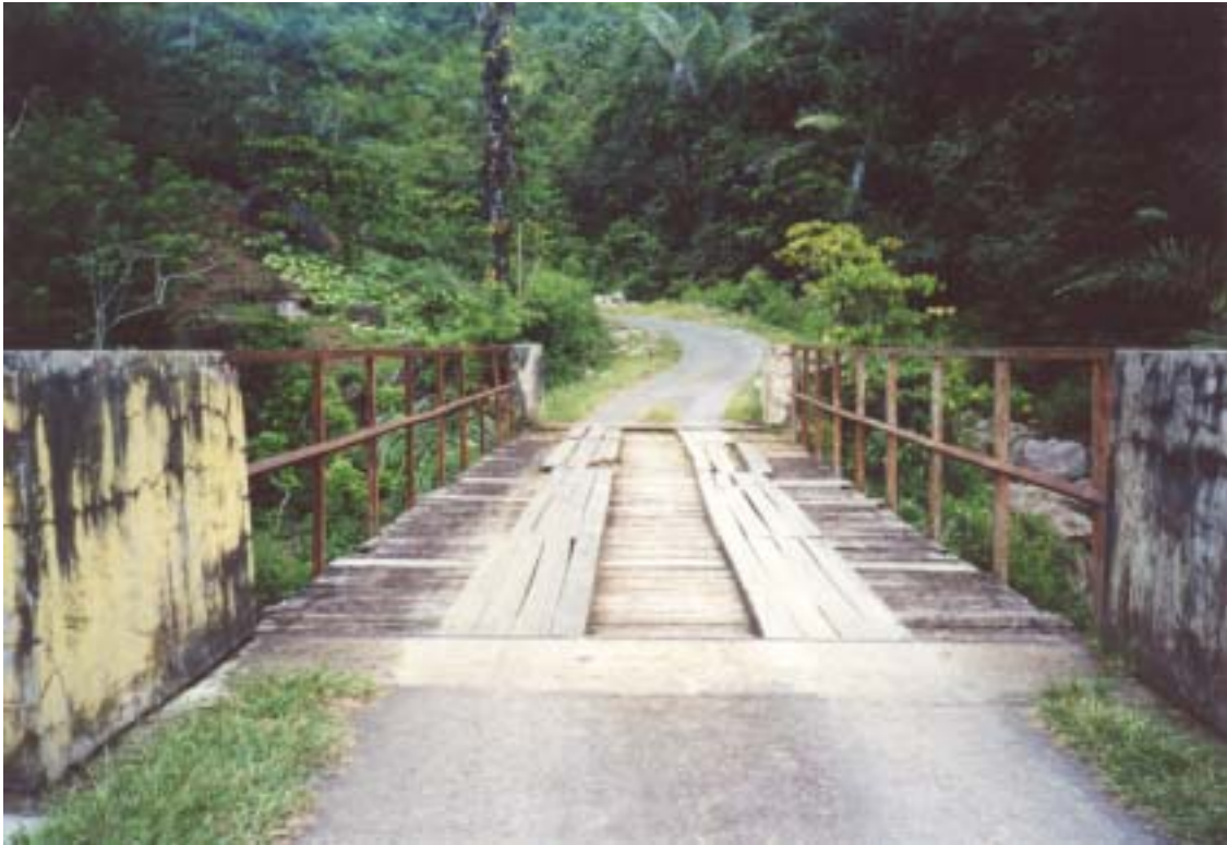
View of bridge showing the timber decking
