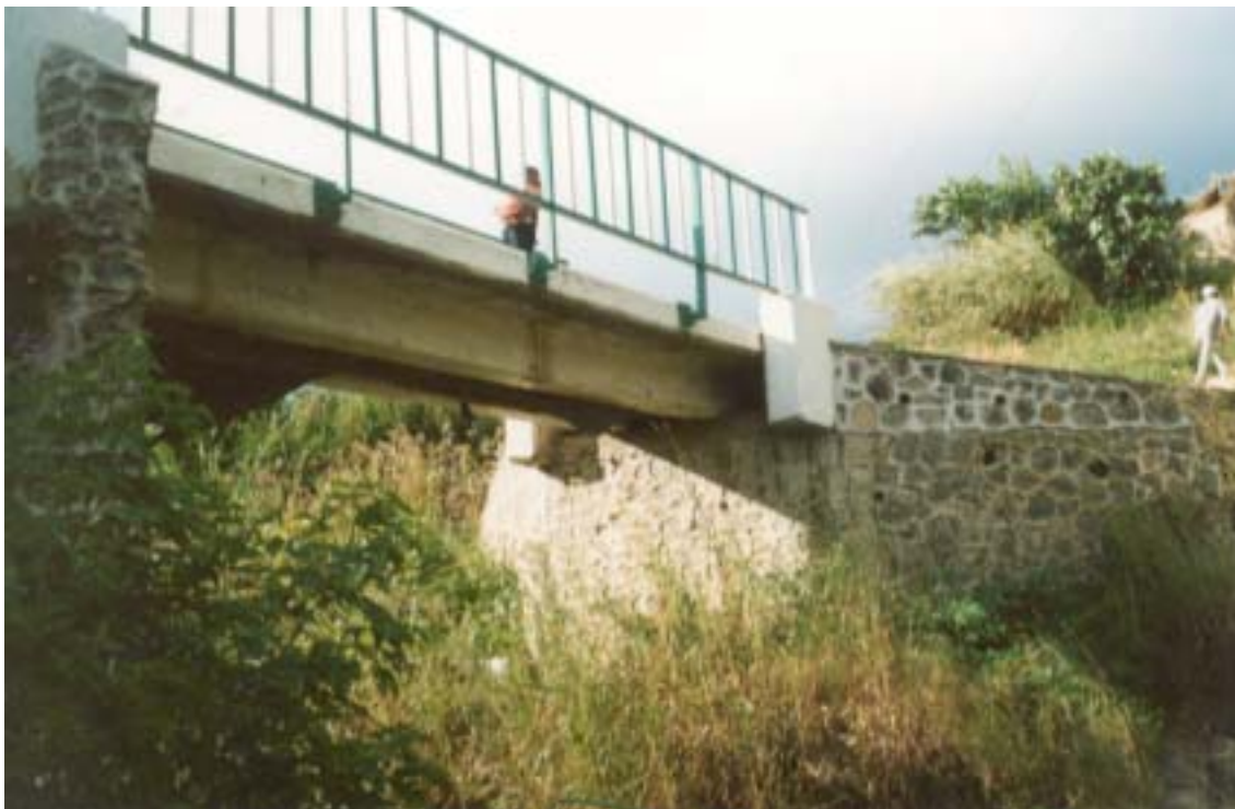
View from Below Showing Integral Beam Reinforcement and Central Pier
