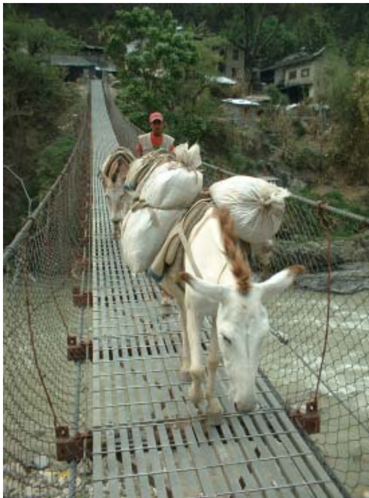
Figure 3.16: Example of a Suspended Footbridge in Nepal (Photograph provided by Chris Rollins, Bridges to Prosperity Inc.)
