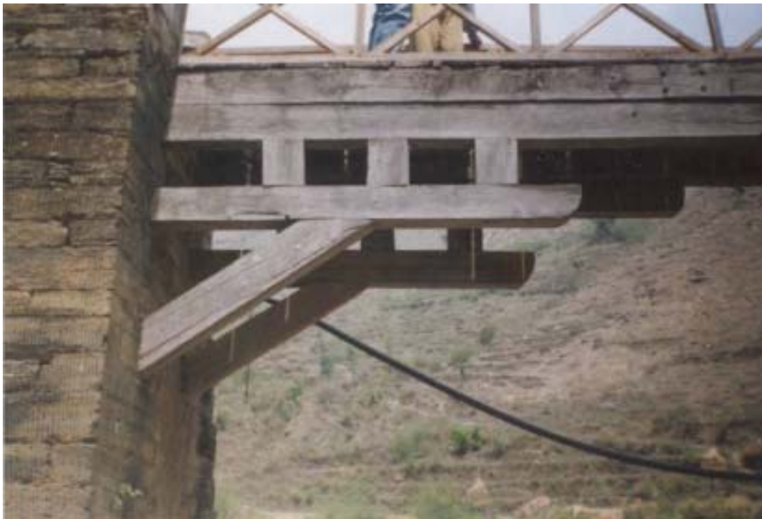
15m span x 1m wide sawn-timber footbridge for pedestrians and livestock. Note the cantilever supports used to extend the single span of the bridge.
