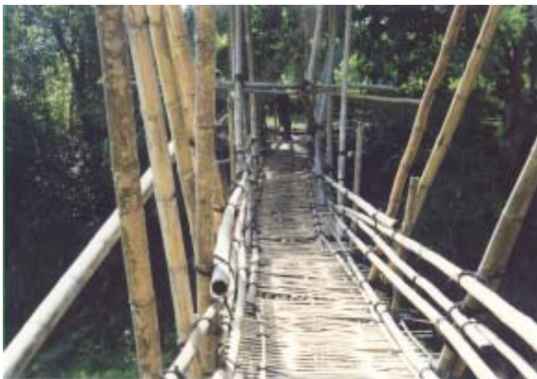
Figure 3.1: Suspended Bamboo Footbridge
