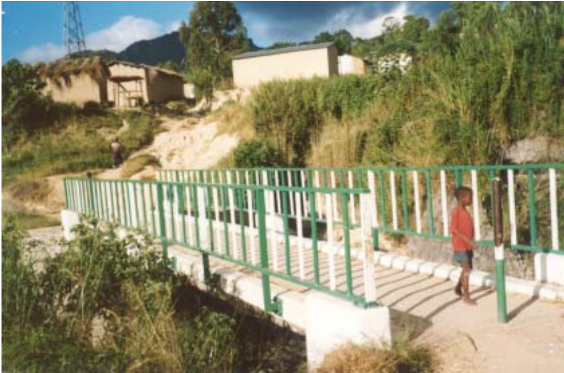
View Showing Details of Bridge and Handrail
