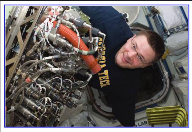
**FIG. 4.** In October 2010, aboard the ISS, NASA astronaut and Expedition 25 commander Doug Wheelock installed the Sabatier system, which extracts more water out of the ISS atmosphere. Sabatier creates water from the by-products of the station’s OGS and Carbon Dioxide Removal Assembly. Image Credit: NASA.
