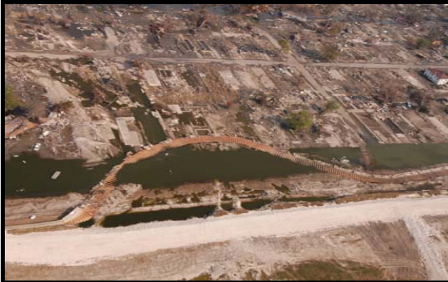
Sheetpile Floodwall Collapse
