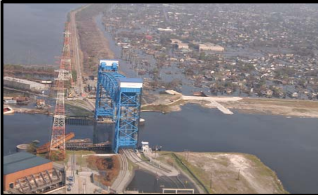
Northern 9 th Ward Breach
