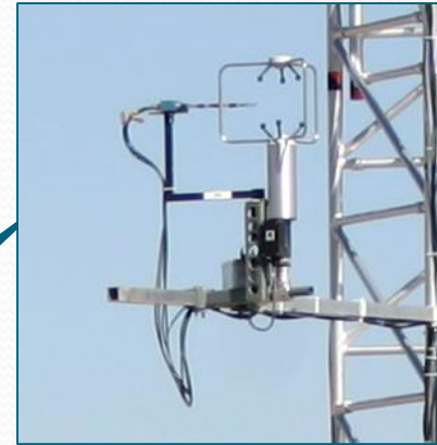
Combo probes located at 2m and 6m
