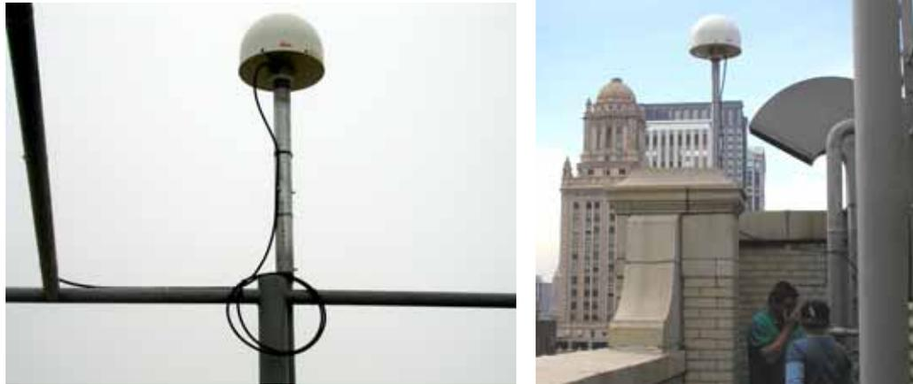
FIGURE 13.3. Fully installed GPS antennas at Building 1/rover site (left) and reference site
