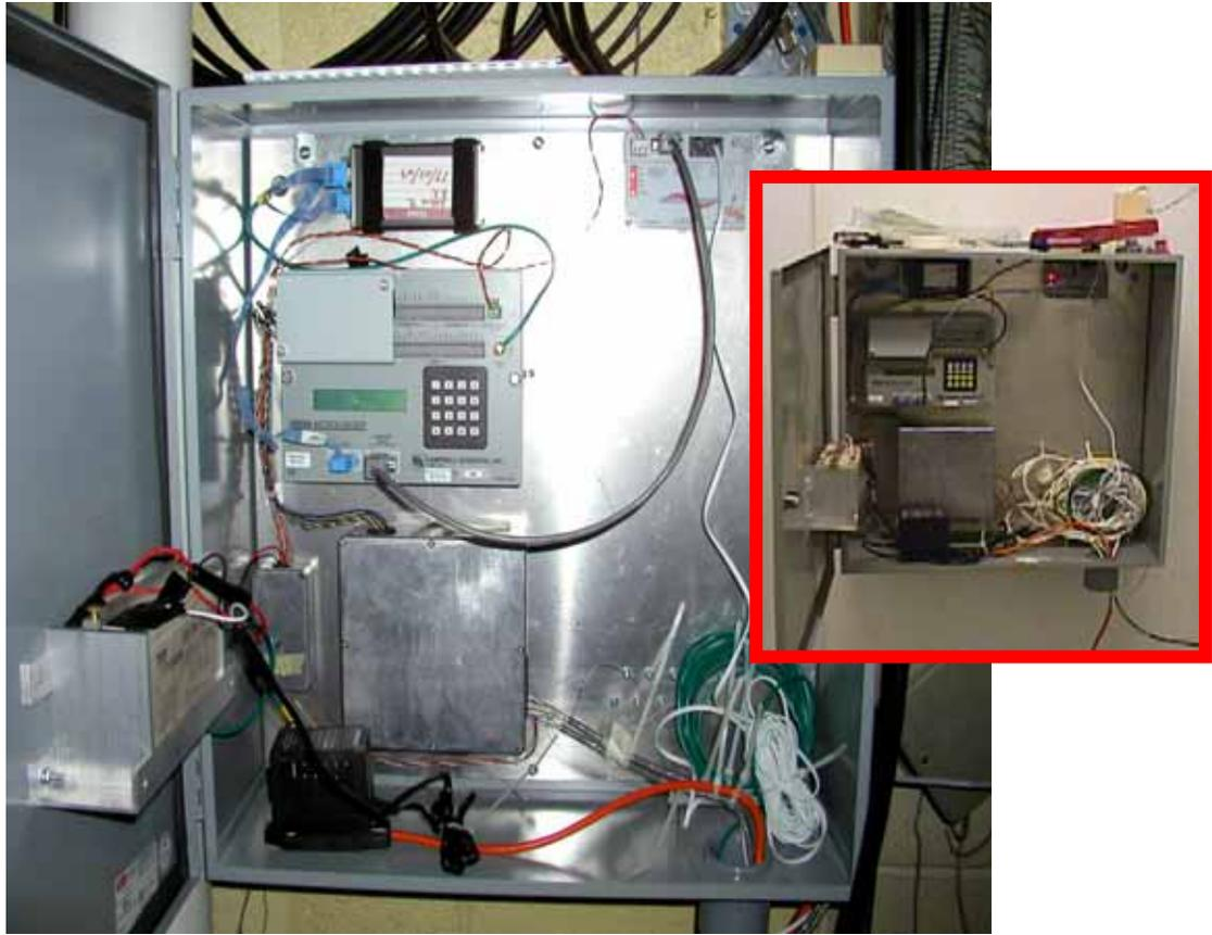
FIGURE 9.4. Data logger cabinet assembly installed in Building 1 (zoomed in for detail) and comparable logger assembly for Building 2 (inset at right)
