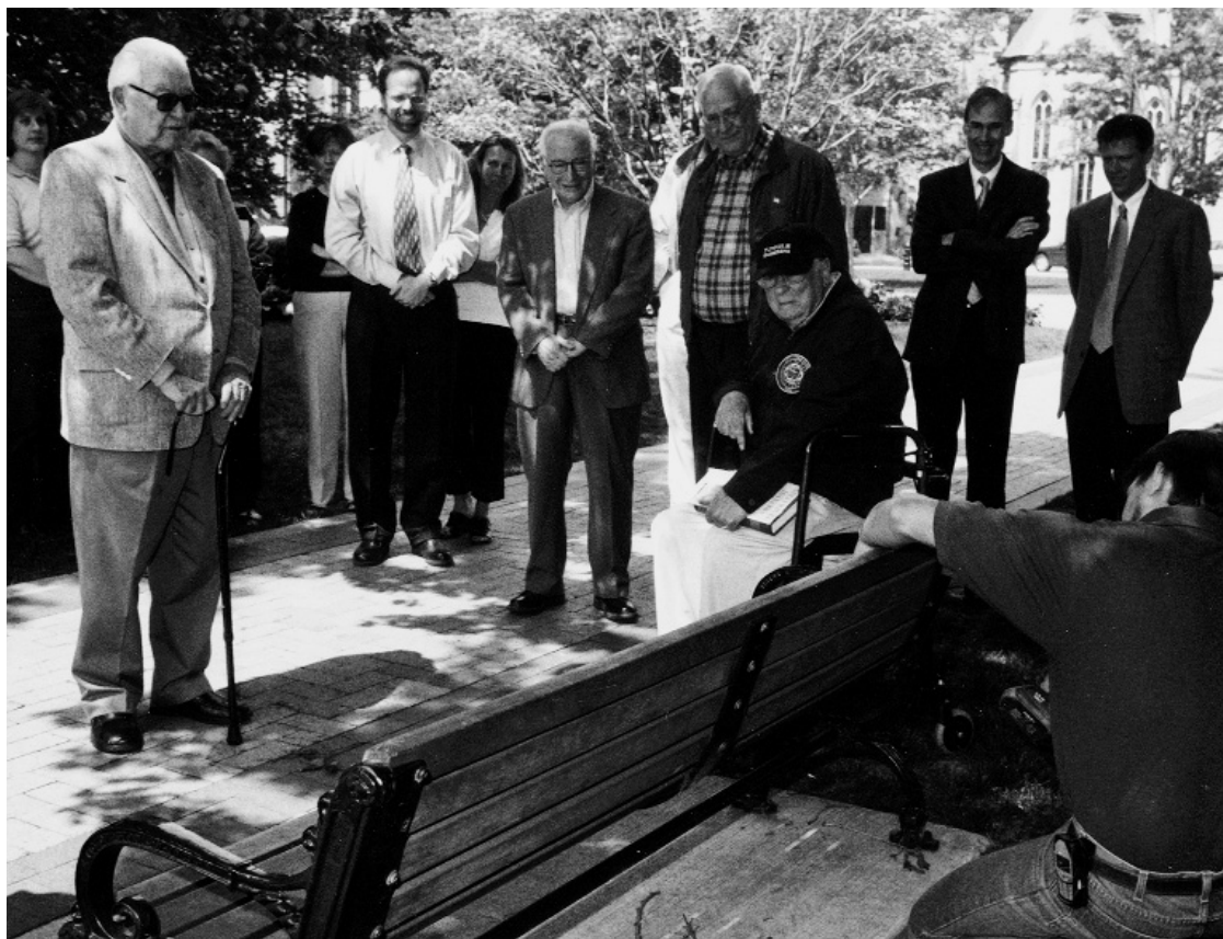
University carpenter Jeff Hojnacki installs the bench slat bearing a commemorative plaque as Emil T. Hofman, seated, President-emeritus Rev. Theodore M. Hesburgh, C.S.C., and an appreciative collection of former colleagues look on. Photo by Lou Sabo.
