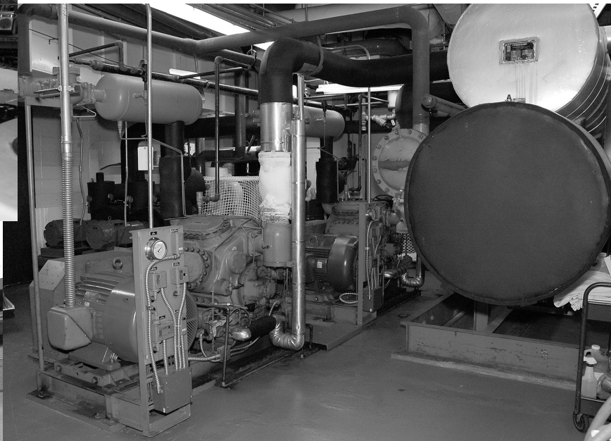
Motorized pumps circulate refrigerant and antifreeze to maintain the ice at 12 to 14 degrees—the heat of the machinery makes the refrigeration room the warmest spot in the rink.
