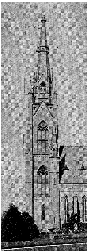
This illustration from the Scholastic Magazine of Sept. 16, 1899 shows Jerome Green's transmission wire hung from the steeple of Sacred Heart Church. Photo provided by Elizabeth Hogan, University Archives.
