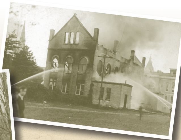
A phosphorous fire broke out on the third floor of the Institute of Technology, which housed the departments of chemistry and pharmacy, on Sept. 13, 1916. Although the fire was extinguished, the chemical spread throughout the building and reignited a week later, starting a fire that gutted the building. The building was dedicated as the Hoynes College of Law in 1919; in 1976 the building, renovated and renamed Crowley Hall, became home to the Department of Music.
