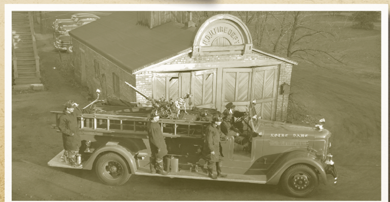
The Notre Dame Fire Department—including "Notre Dame Belle," the company's dalmatian, pose in front of the 1896 firehouse, which stood directly behind the Main Building. The current firehouse was built in 1945, and the old building was demolished.
