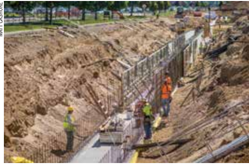
Utility tunnel construction
