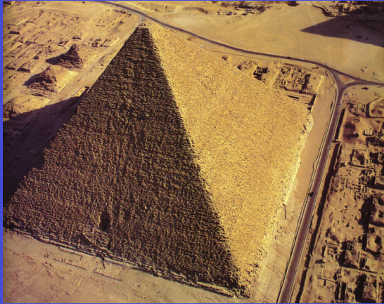
Great Pyramid of Khufu, Giza, Egypt (Old Kingdom: 2686-2181BC). Angle 51^{\circ}52' 146 m high, 2.3 million stone blocks, each 2.5 tonnes. Base is almost perfect square, 229 m sides. Aligned perfectly with cardinal points (N,S,E,W)
