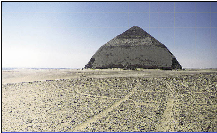
Bent Pyramid at Dahshur, Egypt, 2680-2565 B.C Angle changes from 54 to 43 degrees (foundation/stability problems?). If it had been completed to original plan, it would have been the biggest pyramid in Egypt.
