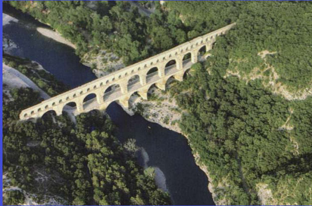
This aqueduct, over the river Gard, is 275 metres long and 49 m high. Part of an aqueduct nearly 50 km long that supplied Nîmes with water. On its first level it carries a road and at the top of the third level, a water conduit, which is 1.8 m high and 1.2 m wide and has a gradient of 0.4 per cent.
