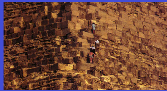
Climbers on the Great Pyramid at Giza (note sizes of blocks) Originally, smooth surface - faced with limestone - now weathered away
