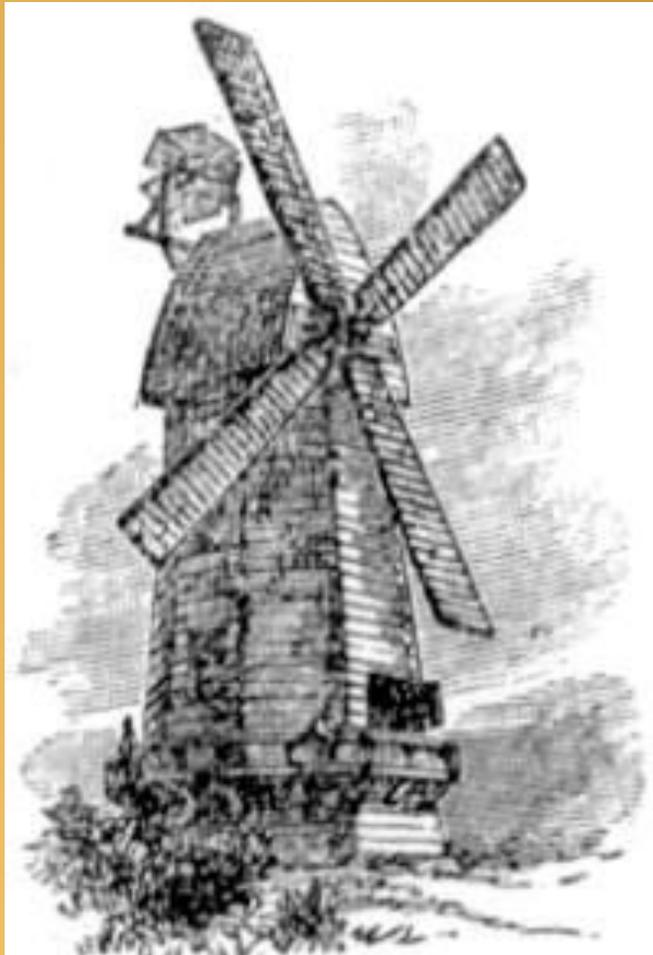
This design incorporated blades attached to a horizontal shaft that used a wooden cog-and-ring gears to translate the motion of the horizontal shaft to a vertical rotation of the grindstone. The miller could manually rotate the post mill into the wind.
