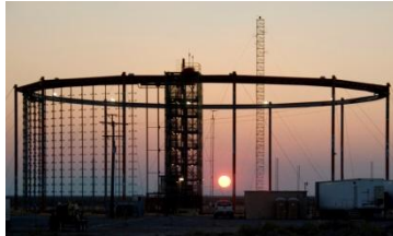
Infrastructure in place with state-of-the-art equipment
